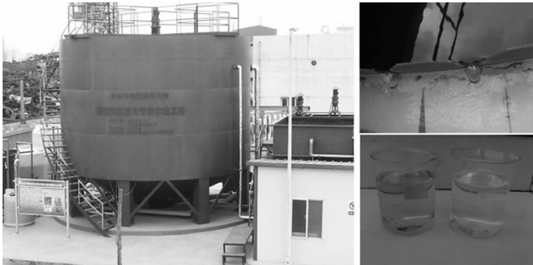
图 25 某纺织产业园区 3600m 3 /d 示范工程现场照片 Figure 25 The photos of 3600m 3 /d demonstration project for a textile industrial park
