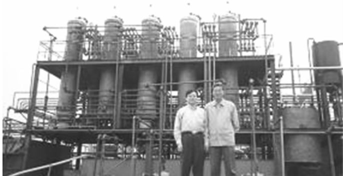
图 8 苏州迪通化工有限公司废水处理设施 Figure 8 Wastewater treatment facilities of Suzhou Ditong Chemical Co. Ltd.
